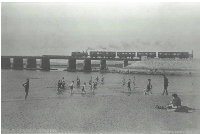
Figure 14: Arnside Railway Viaduct
