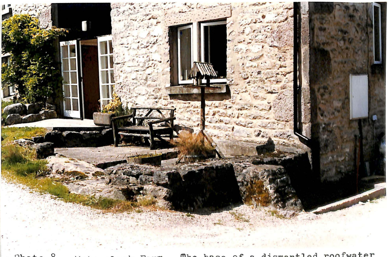
Photo 8. Waterslack Farm. The base of a dismantled roofwater storage tank, later adapted as a farm building, and now a sitting-out area. The trough to the right was filled from the tank, to water farm stock.
