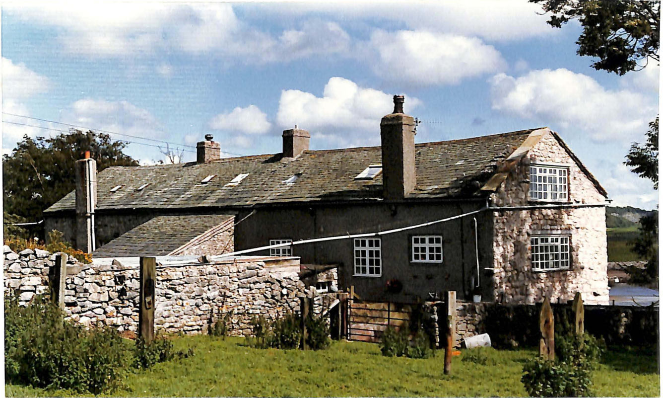
Photo 12. A roofwater supply system still in use at Brown's Houses, Silverdale in 1993. Water from the front half of the roof (on the right of the photograph) is brought across the gable end to join water from the back half of the roof. This is carried across to a tank in the back garden. Additional rainwater is collected from the metal covering on the tank.
