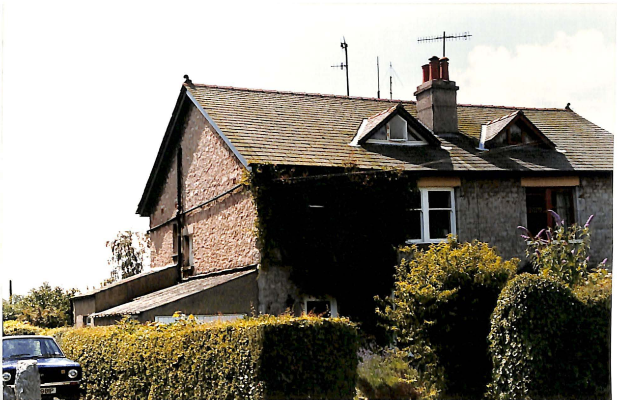
Photo 7. Gutter on the gable-end of a house in Cove Road. The gutter is still in its original position, designed to carry water from the front roof to a storage tank at the back of the house.
